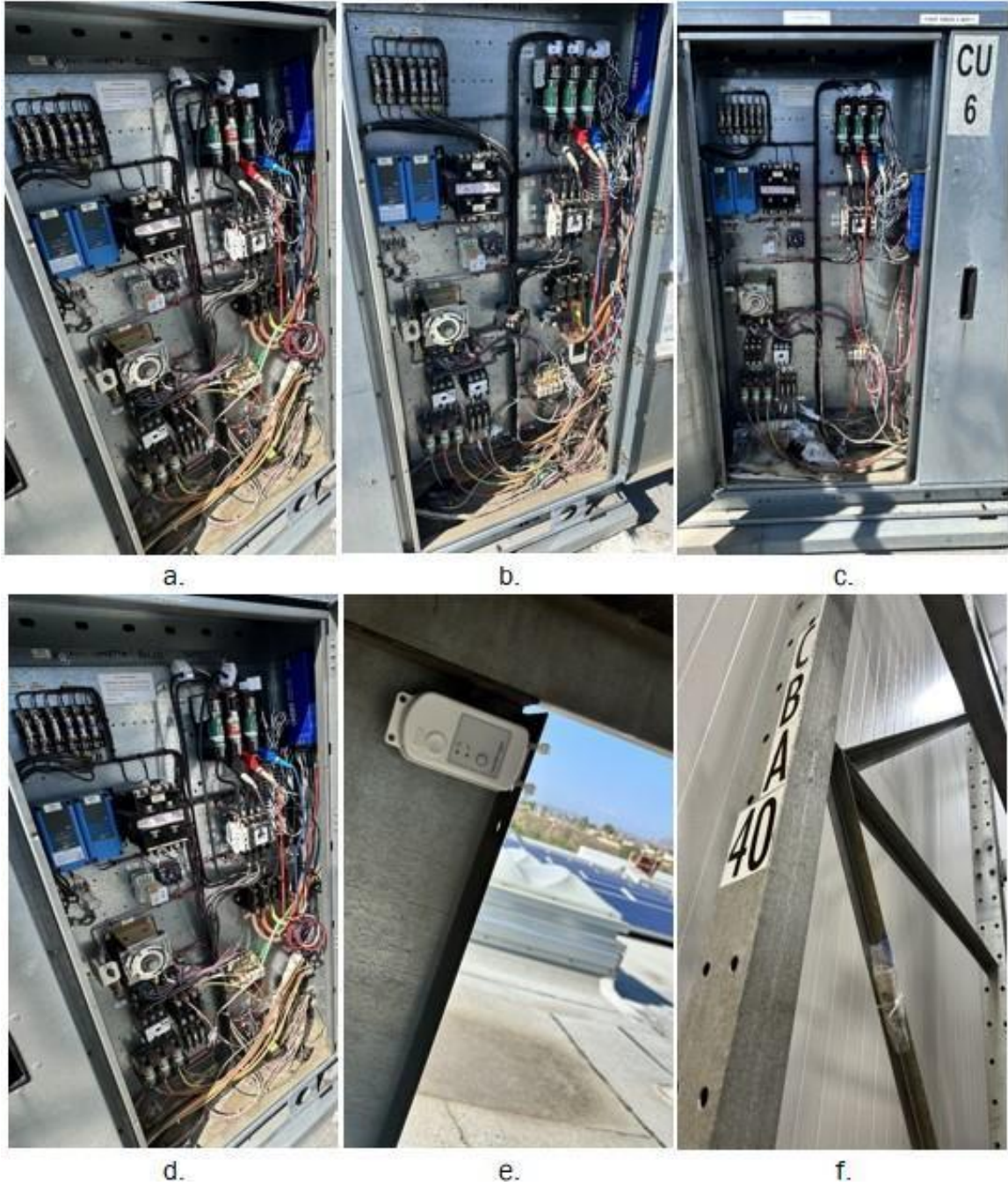
Figure 27: DENT logger with CU5 east (a), DENT logger with CU5 west (b), DENT logger with CU6 east (c), DENT logger with CU6 west (d), OAT logger (e), and space temperature logger (f).
