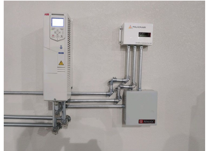
ABB VFD with SCC at Roessler
