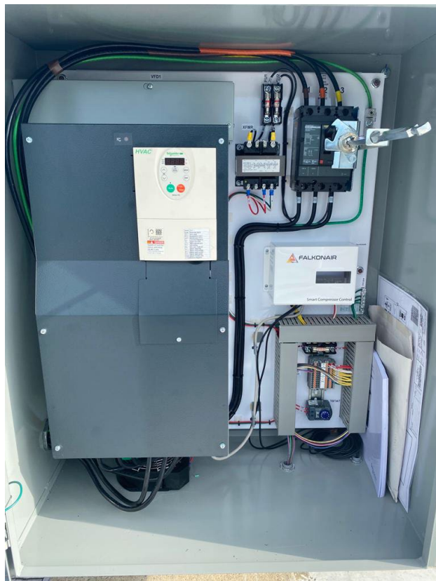
Schneider VFD with SCC
